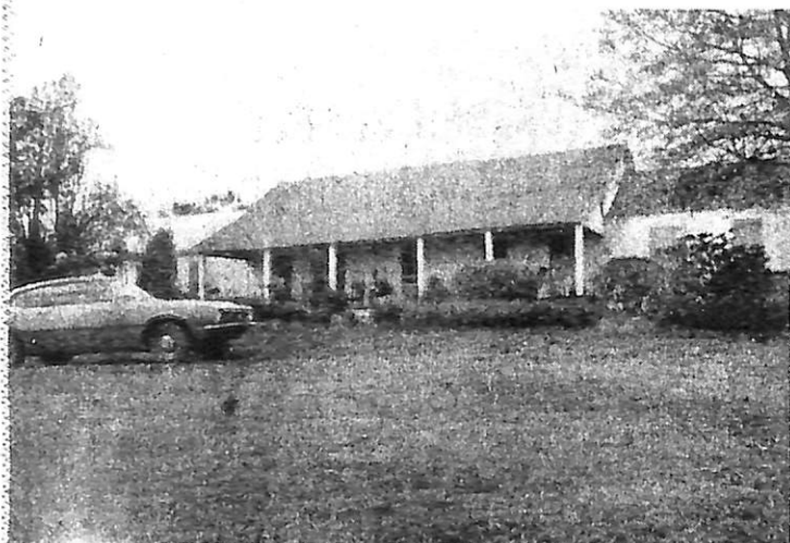
STORM DAMAGE REPAIRED - The roof is back in place after last years tornado damage at the 140 year old home owned by Mr. and Mrs. Claude Marshall at Little Yazoo.
