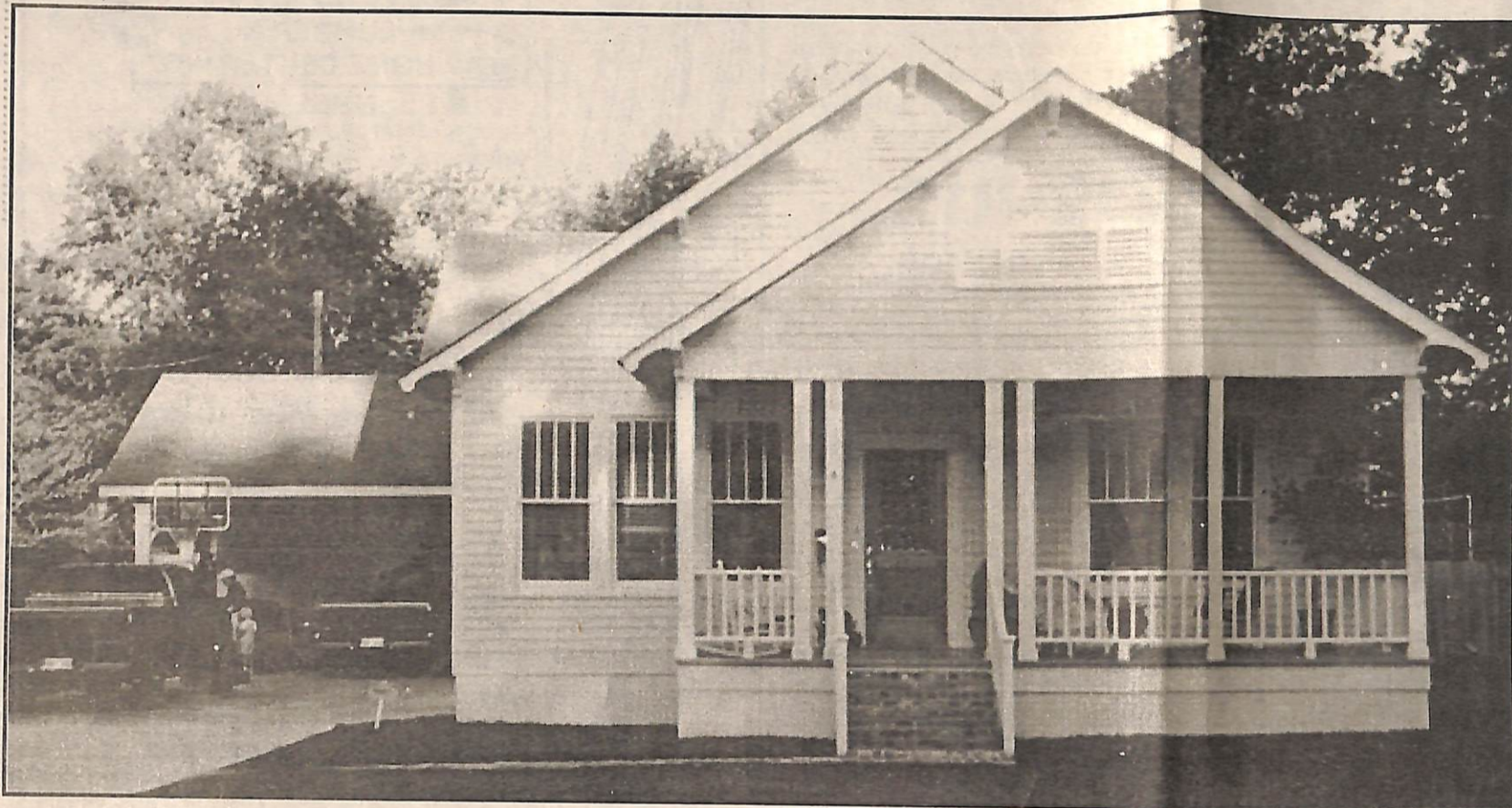
The Billy Brown Jr. home after extensive renovation and remodeling
