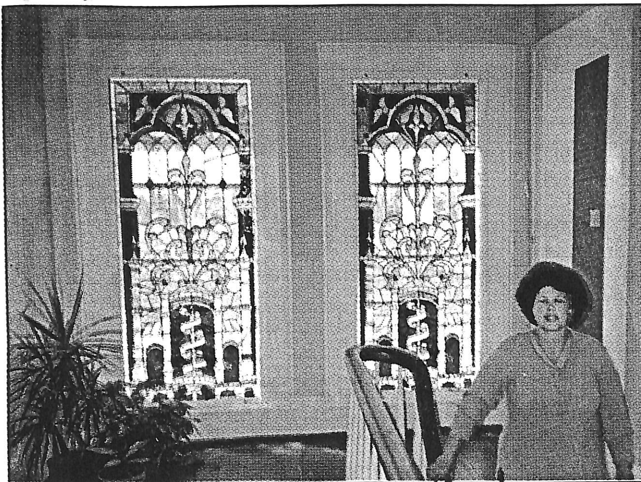
ON THE SECOND FLOOR LANDING, STAINED GLASS WINDOWS now enclose the west side of the once-open back porch. One of the few details added to the structure by Janet Whittington in the restoration, the windows featured colors which repeat those of the original glass around the second floor, front porch door.
