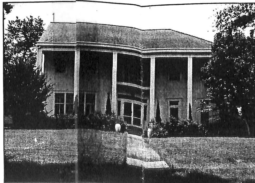
WOODBINE, CIRCA 1942. Barely visible at bottom left, a one floor wing has been added to accommodate additional family during the Depression. The front doors have been replaced and screen doors added. Also, the top veranda has been removed and the landscaping changes again.
